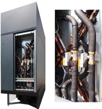
Water flow control valve section
